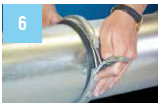
6 Snap QF Clip over O-ring and one end of slip duct.
