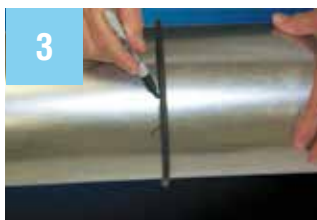
3 Use O-ring provided and mark for cut.
