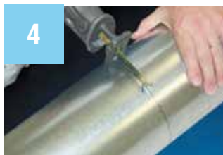
4 Drill access hole(s) and then cut the duct.
