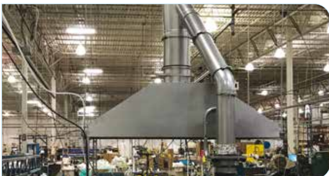
An example of Transition from rectangular to round.
