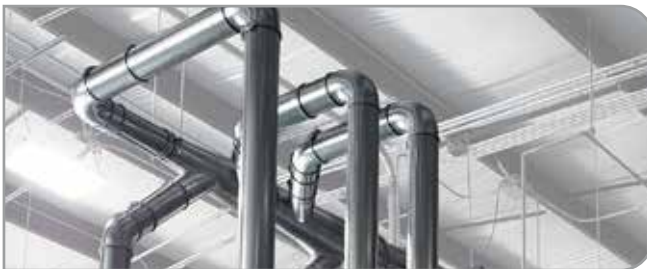
Quick-Fit Duct System installed.
